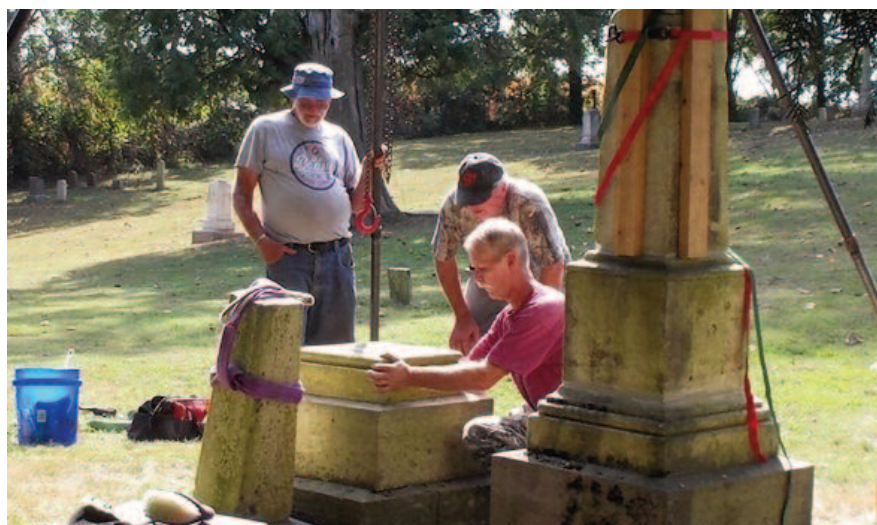
From left: Dave Nicols, Greg Drennen and Mark Morton use a 14-foot tripod to set one of four obelisks at Capitol Hill Cemetery in Cambridge City, Indiana. (Photo courtesy of Cynthia Nicols)
