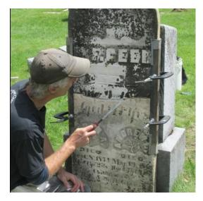
After the crack has been cleaned of epoxy, and the color block of correct material has been matched to the stone. It is time to mix a batch of infill material. Check the infill material list for recommended material.
