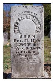
When ready to infill, use a misting bottle and dampen the stone (not dripping wet) so the mortar will stick to it (mist more as you work if it starts getting dry). Using a small thin trowel, push the mortar into the cracks and voids, making sure to fill it in well. You should use gloves, but I like to 'feel' what I am doing so I don't use them. I also tend to use my hands instead of the fine trowel to push the mortar in.
