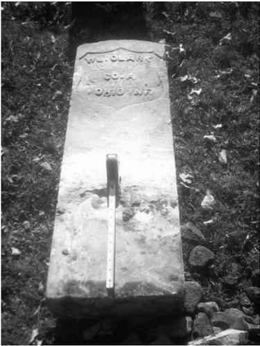
Once you have removed the stone and secured it and your equipment safely, you can begin work on the new hole. You first have to determine the size and depth of this hole. This takes us back to the rule of 1/3's and measuring the stone to find out what that figure is.
