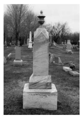
Obelisks (photo C) as well as larger, thicker tablets can be set onto a base (photo D).
