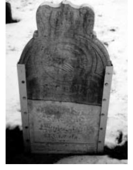
Drilling through a marker to affix braces is never an acceptable alternative.
