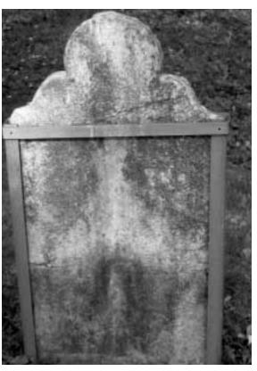
In rare circumstances, unorthodox repairs such as this application serve its purpose. The metal braces used are stainless steel and do not restrict movement of the stone while it still holds the marker upright.
