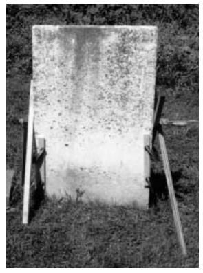
After the repair has been made, securing the marker is imperative. The use of clamps, wooden braces and shims assures the marker is not touched by the metal clamps, and also prevents the marker from moving while the repair treatment cures.
