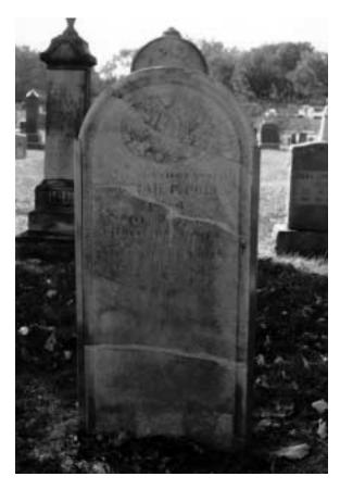
Professional conservators have in unique situations, girdled a marker with stainless steel channel. Here the repair is not easily seen and has not compromised the stone.
