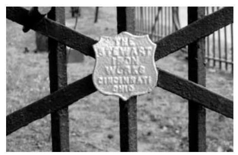
In some instances the original company nameplate will remain on the wrought iron fence. This information is valuable when trying to replace or repair fence sections.
