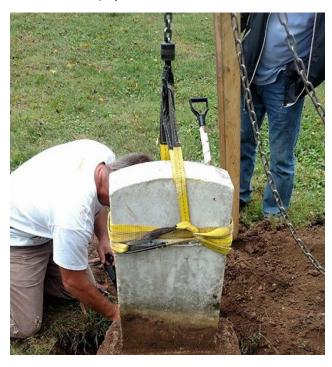
The strap and hoist method is the safest and most supportive for the stone. As seen in the video below. This method will require a 1 ton hoist and a tripod or gantry to attach it to.
