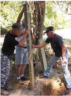
Some tablet stones can be quite tall and heavy and require extra care and assistance for safety sake as well as ensuring no damage occurs. The larger the tablet, the more support is required.
