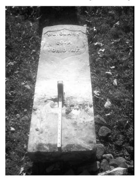
Once you have removed the stone and secured it and your equipment safely, you can begin work on the new hole. You first have to determine the size and depth of this hole. This takes us back to the rule of 1/3's and measuring the stone to find out what that figure is.
