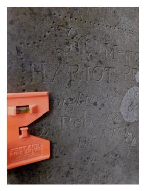
Now you are ready to place the stone in the hole. When this is done you will want to check your desired row alignment and begin to level the stone. A post level is the best tool for this because it will easily allow you to check square-ness in both directions at once. You want to be both plumb and level.
