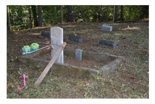
Repaired headstone and foot stone returned to the concrete enclosure. Repaired, plumbed, and standing tall.
