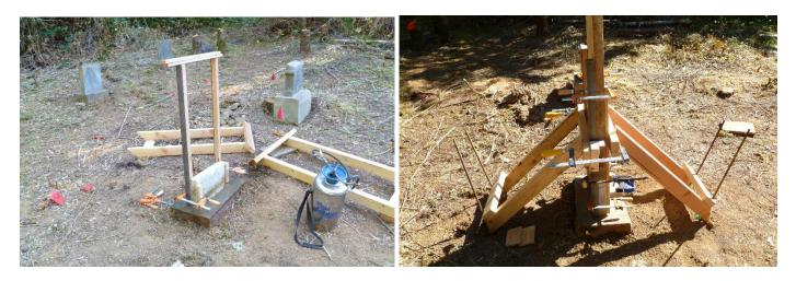
The second type of broken headstone is where the bottom section will not provide sufficient support for the top while the epoxy cures without using external bracing. The top of the headstone is much larger than the remaining piece in the slotted base.
