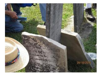
After this stone was evaluated and deemed to have no serious delamination or issues of sugaring, it was carefully excavated for cleaning and prep. It was cleaned with D/2 and left to dry thoroughly in the sun. Epoxy should only be applied to dry stones. The edges at the break were gently wire brushed to remove any leftover loose dirt that would adversely affect the epoxy bond. Mendable edges like these are the ONLY areas you should ever use a wire brush on.
