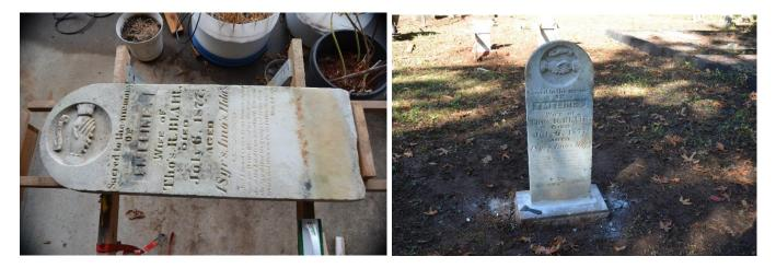
The picture above is the finished headstone. The voids were filled with a mixture of white Portland Cement, lime, fine white sand, and colored to closely match the stone. Your void fill mixture may be different but some have to follow the state guidelines. As you can see from the picture, some of the staining was not removed. D/2 will work over time so hopefully more of the stain will disappear. The
