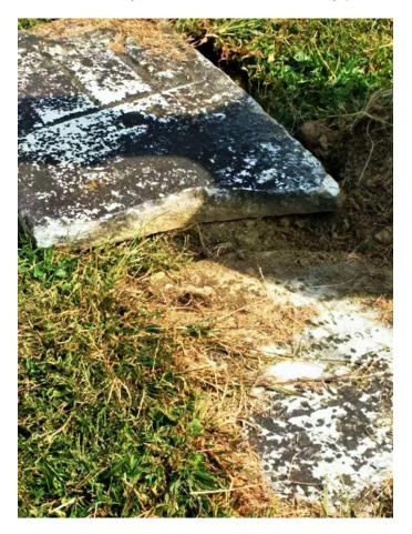
Tablets in the condition like the one to the left are quite common. This is a white marble tablet that fits into a slotted base and has a single break. This tombstone was chosen to demonstrate how to repair a single break at a cemetery preservation class.
