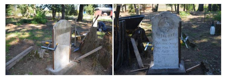
For this type use the angle braces and clamp them to align the top to the bottom of the headstone. Ensure the edges and the faces of the headstone are aligned. Make a test fit before you epoxy the pieces together. This will allow you to see where the epoxy should be placed and ensure proper alignment of the broken piece.
