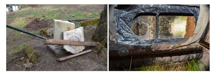
A headstone broken into two pieces with bottom set in a slotted base, and a headstone that was broken into two pieces and no longer attached to its' slotted base.
