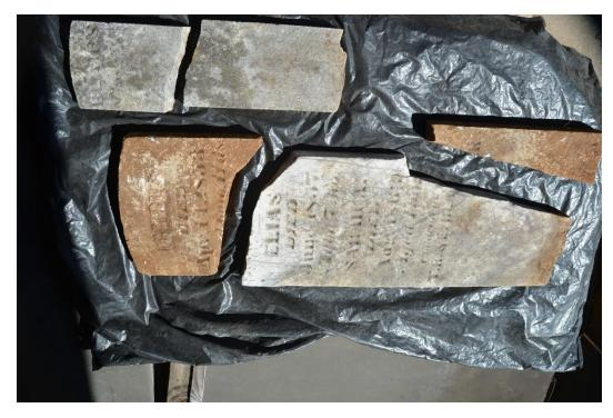
These multiple breaks consist of a headstone that was broken into three pieces, no longer in a slotted base and a footstone in two pieces.
