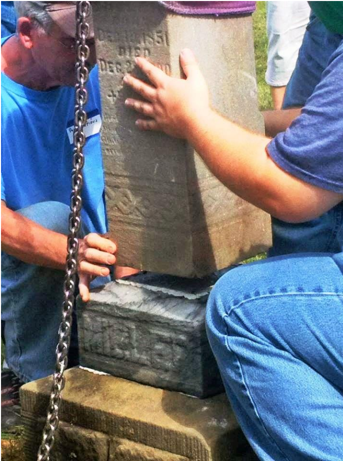
Setting the top obelisk type piece straight down using mortar and setting compound.
