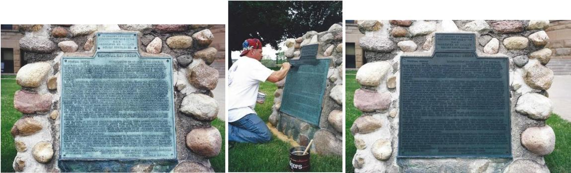
In the pictures above, Brad again adheres to this principal of keeping it simple in a do no harm manner by simply cleaning and waxing this placard.
