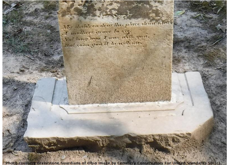
Photo courtesy Gravestone Guardians of Ohio Image by Cemetery Conservators For United Standards 501(c)(3)
