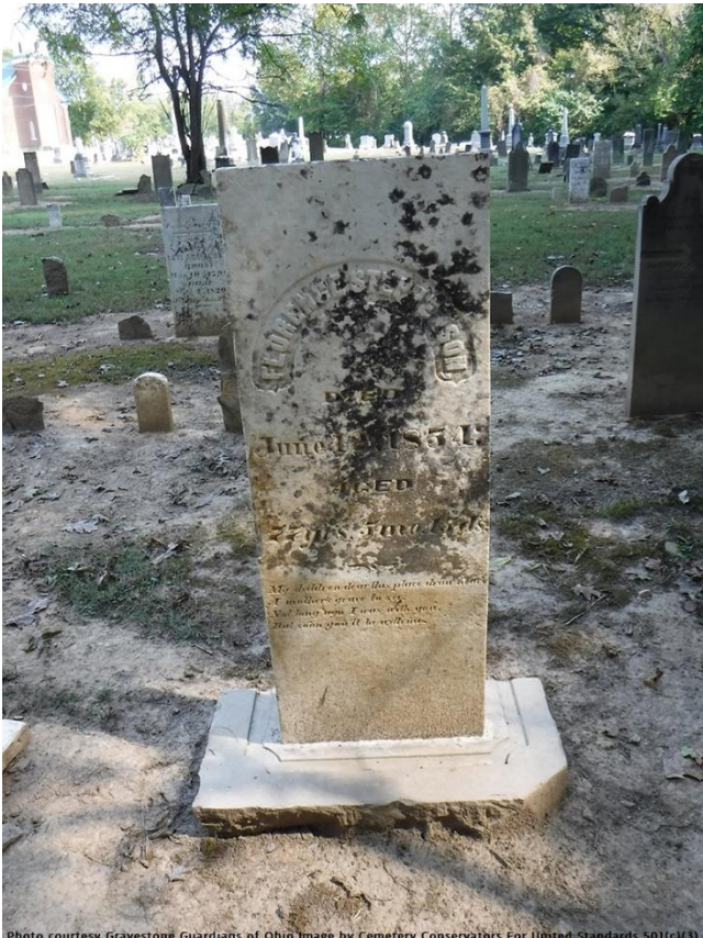
Photo courtesy Gravestone Guardians of Ohio Image by Cemetery Conservators For United Standards 501(c)(3)
