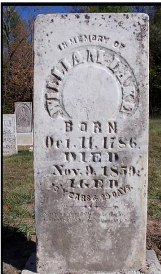
When the cracks and voids are filled to my satisfaction, I use my fingers to feel and make sure it is flush with the surface of the stone. Using a triangular makeup sponge, I get the sponge wet and then squeeze out the excess moisture and then draw it lightly across the mortar and stone, 'feathering' the finished edge.
