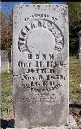
When ready to infill, use a misting bottle and dampen the stone (not dripping wet) so the mortar will stick to it (mist more as you work if it starts getting dry). Using a small thin trowel, push the mortar into the cracks and voids, making sure to fill it in well. You should use gloves, but I like to 'feel' what I am doing so I don't use them. I also tend to use my hands instead of the fine trowel to push the mortar in.
