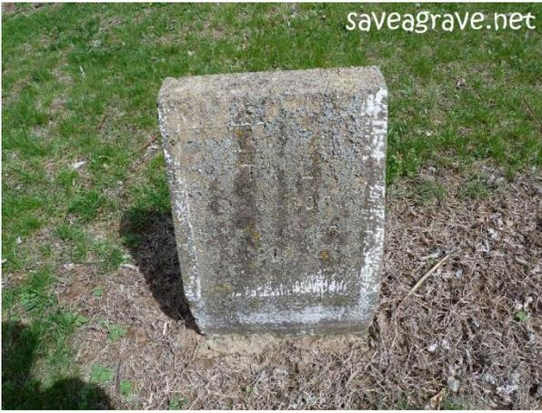
This stone has flaking, only use a soft dry brush to try and clean off some of the flaking before using any method to read the stone.
