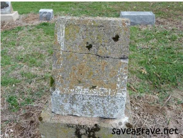
You should not touch a stone like this one. It has been repaired and with any pressure the top could fall off.
