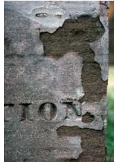
Figure 13. The impervious coating used to "protect" this sandstone grave marker trapped moisture within the stone, eventually resulting in deterioration and surface loss. Photo: Fran Gale.
